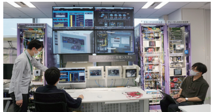
The simulated plant used for Testing
