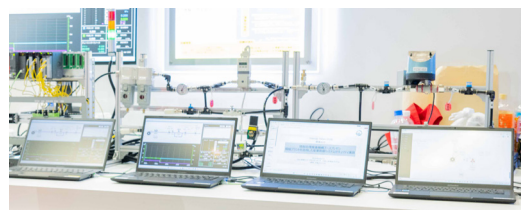
Simulated gas supply plant and HMI screen
