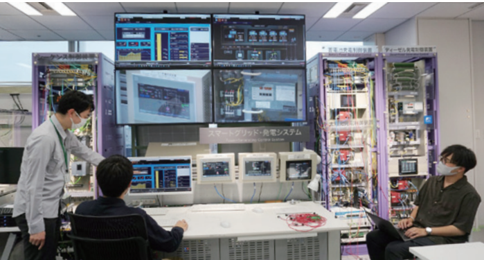
The simulated plant used for Testing
